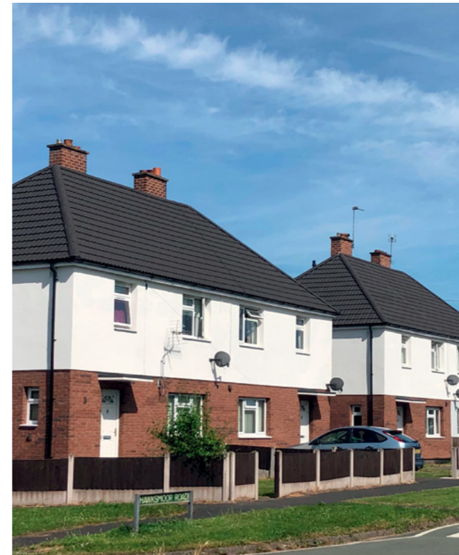
Stafford & Rural Homes Basic 1 & Basic 4 Systems consisting of 100mm EPS insulation boards. The ground floor area makes use of acrylic brick slips, while a Silitect T 1.5 finish has been applied to the first floor.
