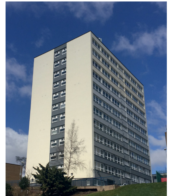
Bucknall New Road Ecomin 300 & Ecomin 400 system consisting of 100mm Ecomin insulation boards with Staffordshire blue clay brick slip to ground floor. The first floor up boasts a gradient effect in an array of cream and grey colours created using a silitect T 1.5 finish.
