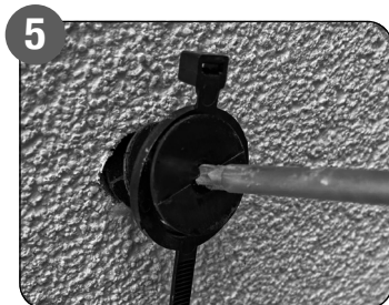
5 Insert the spiral into the pilot hole, and using a PZ2, gently screw the spiral into the EWI system.
