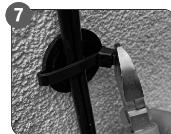
7 Remove any excess length of cable strap.
