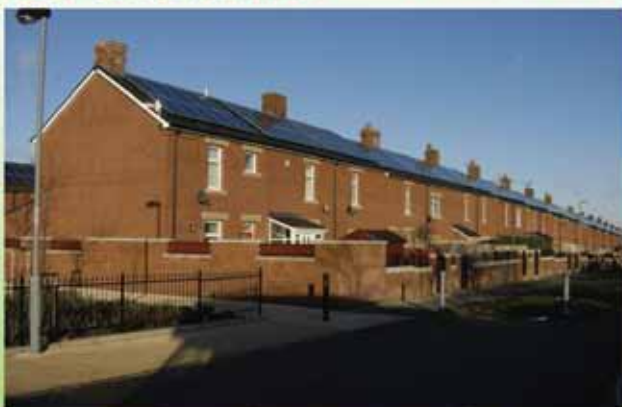
Shaded Brick Render & Feature Stonework, Craghead, Co. Durham.
